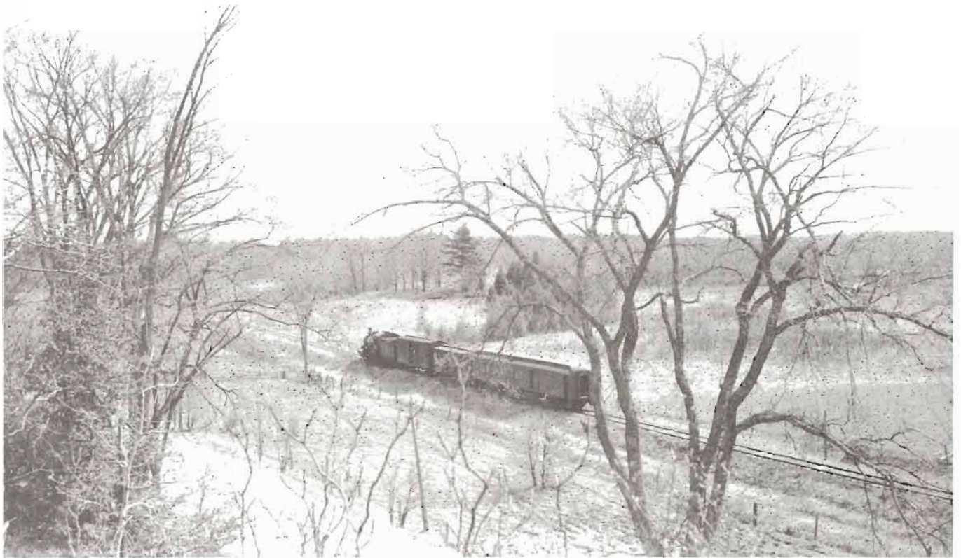
No. 340 has just rounded a curve near Delta, Ontario, and passed a Canadian Northern feature, a water syphon on a short trestle bridge at mileage 24.10. With its shaky finances, the CNoR frequently opted for syphons as an alternative to the more expensive water tank and pump house. Note how the consist has swelled by one car. Also interesting is the poorly ballasted track, not to mention the untreated ties! (Omer Lavallée Photo, April 1951)
