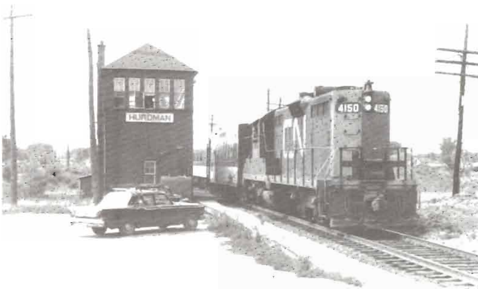
Hurdman Tower sits forlornly October 22, 1966, just two weeks from the date of its burning November 8 by the NCC. In this view looking south, the raised embankment that was built to connect the western end of the station trackage to the former Beachburg subdivision can be seen. To the right of the tower is the location of the former Hurdman Spur. Photo: Bruce Chapman
