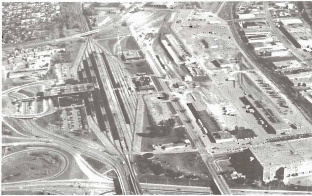
This overall view of the new Ottawa Station shows the entire complex: station, freight terminals, and the main Ottawa Postal Terminal in the right foreground. This mid-1988 photograph shows track 6 full of VIA Rail cars stored out of service. To the left is "Train Station", the bus transitway station which allows passengers direct access to the front entrance of Ottawa Station. Photo: courtesy VIA Rail.
