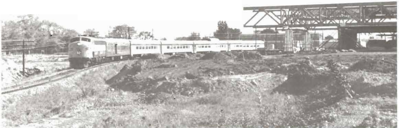
CP train 233 "The Rideau", powered by one of CP's three E8A units, takes the detour or "shoo-fly" track around the construction site of the new Ottawa Station in 1965. In the near foreground can be seen the former CP right-of-way. Photo: Douglas Stoltz
