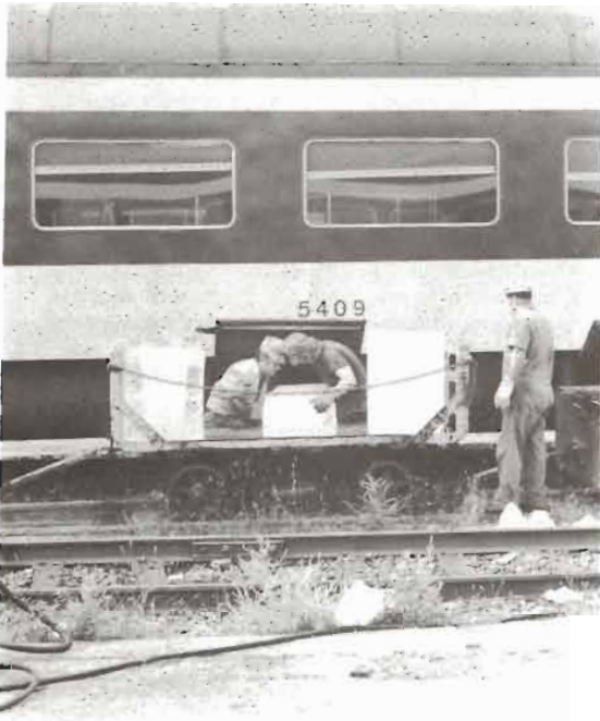
ABOVE: A time-honoured practice of the past. The "Ice Gang" fills the ice bunkers of CN Coach 5409 at Spadina Coach Yard in Toronto, circa 1976. Photo by Brian Westhouse.
