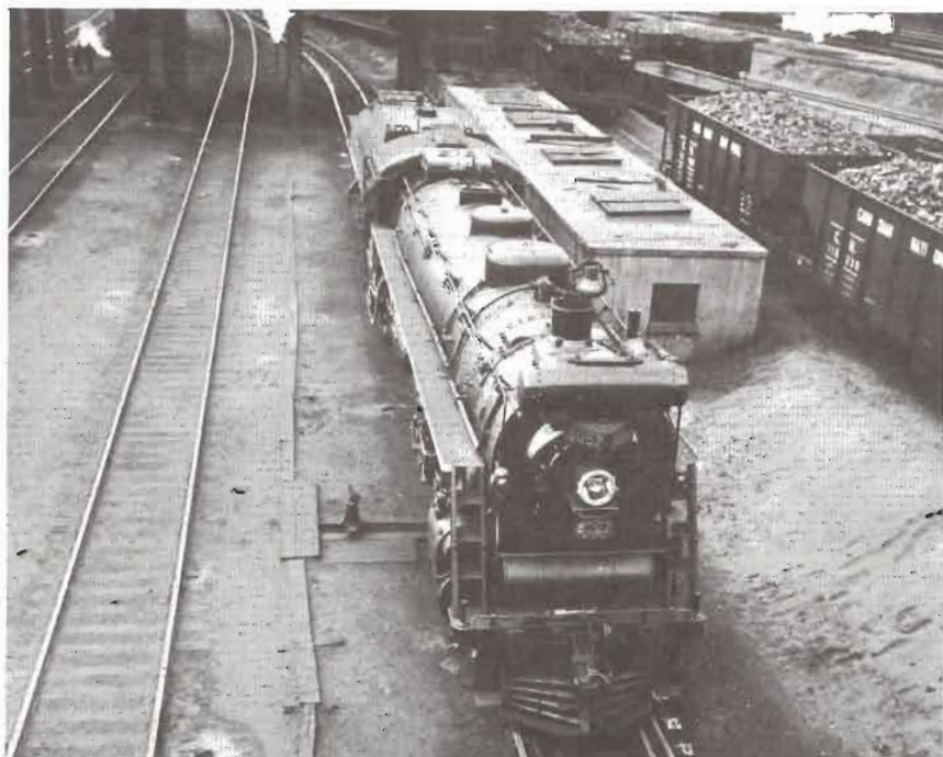
CN 6057 has no need of the coal chute but has stopped for sand at the sandhouse at Spadina roundhouse in Toronto during the summer of 1932. This photograph shows the unusual placement of the bell, as well as the flat surface of the tender oil compartment. CNR Photo 33830.
