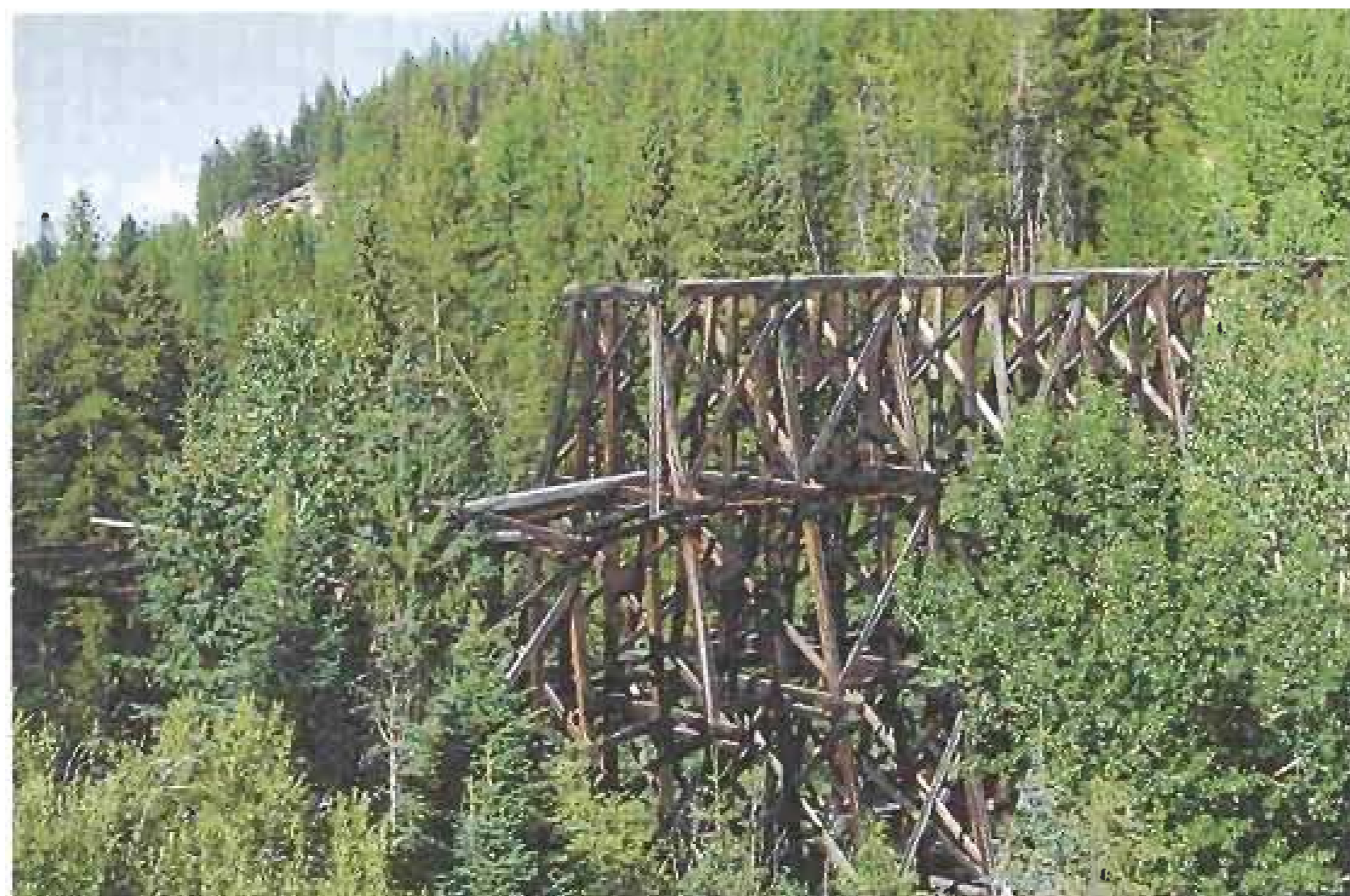
An abandoned trestle in Myra Canyon.
