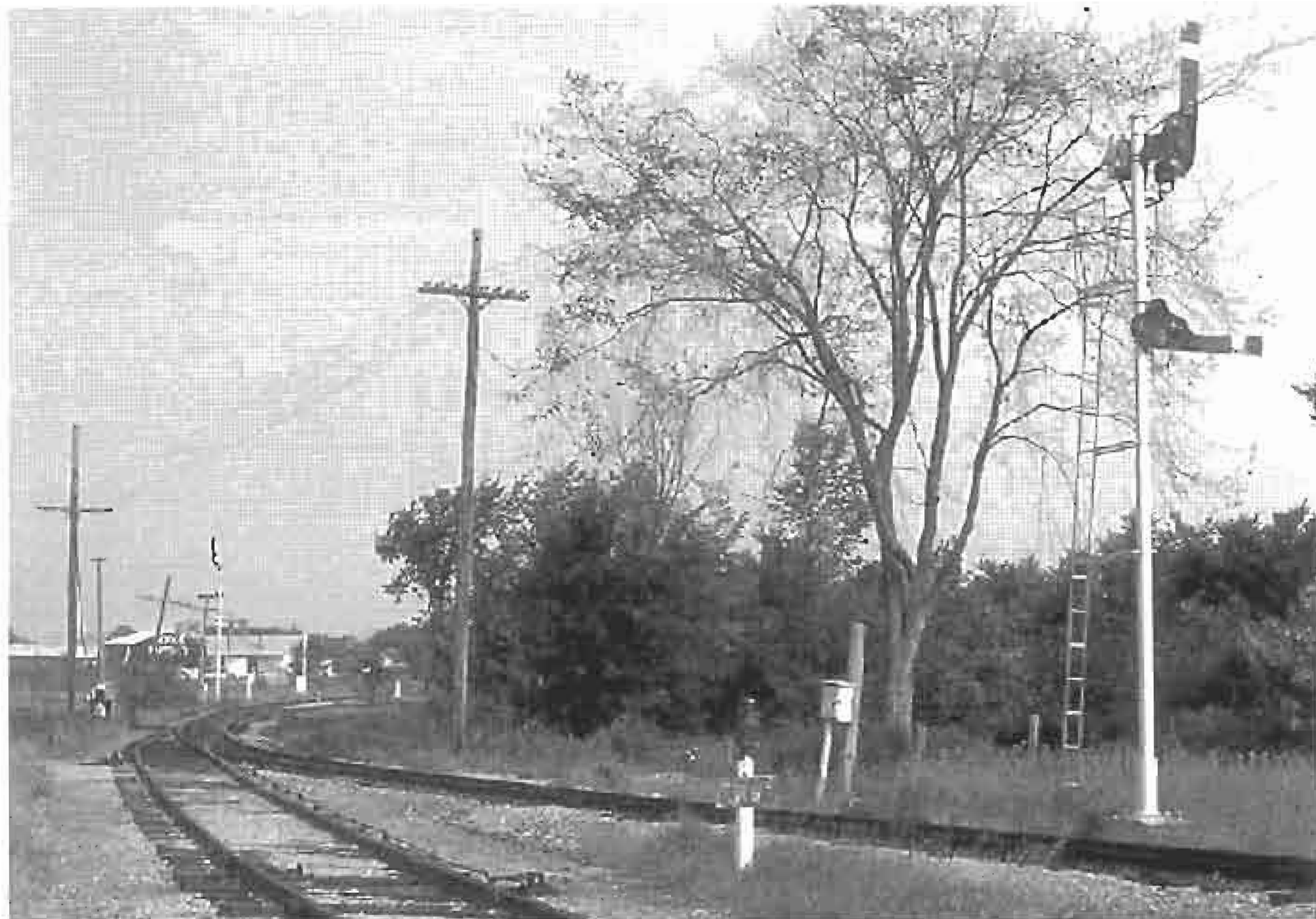
Semaphore signals guard the 'crossing' of CN's Smiths Falls Subdivision and CP's Kingston Subdivision at Harrowsmith, Ontario. According to CP Timetable 48, April 30, 1972, for the Kingston Subdivision, "Jct. with C.N.R. mileage 85.1 - Non Interlocked, switches equipped with electric locks. Rule 104C applies." The semaphores guard the CN track. Note the 'dwarf' signal guarding the CP connection as well as the rodding connected to a derail on the CP side, opposite the dwarf. Years earlier, the junction and crossing were guarded by a manned tower, another story for another issue. Photo by Keith Hansen.
