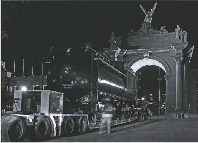
After 49 years at the CNE grounds, 6213's 60-ton (dry weight) tender is the first one allowed to leave. It is poised at the Princes' Gate main entrance, waiting for the streetcar wires ahead to be de-energized and raised to allow passage. The archway width of 25 feet precluded the wider locomotive float taking this direct route out six days later. Photo at 00h58 on June 4, 2009 by Bob Sandusky.
