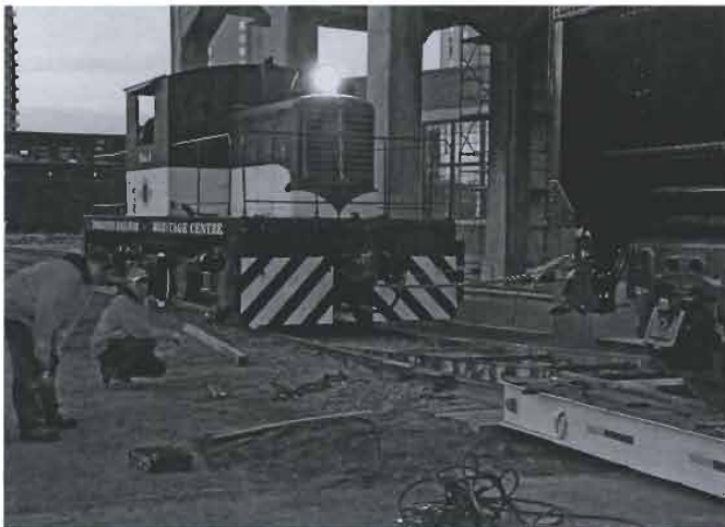
With Toronto Railway Heritage Centre's 50-ton Whitcomb diesel No. 1 chained to one end and a winch cable on the other, 6213's tender is approaching to head down a short and gradual ramp to its new home in what appears to be a simple exercise. The completion of this task took longer than the road move from Exhibition Park due to unforeseen difficulties with the lightweight ramp. It's 05h29 on June 4, 2009. Richard McQuade persevered through the night to record this scene.
