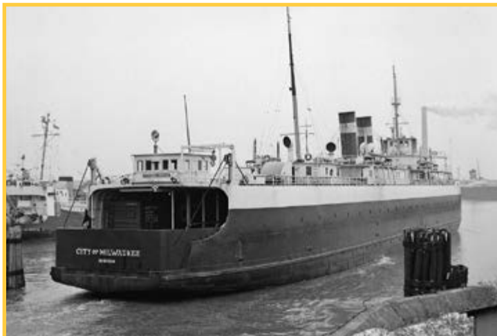
3. Above – City of Milwaukee just pulling out of its Milwaukee slip, January 1966. The sea-gate has already been lowered for the sailing on the lake. A GTW boxcar is on the farthest track at the interior left.
