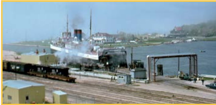
11. Below – Shows the City of Milwaukee after completion of its backing but just before the stern actually nudges the apron that will link it to the shore. There is still a foot or two between them. The gate has been raised for an engine and idlers to unload the boat. Photo taken May 1975.
