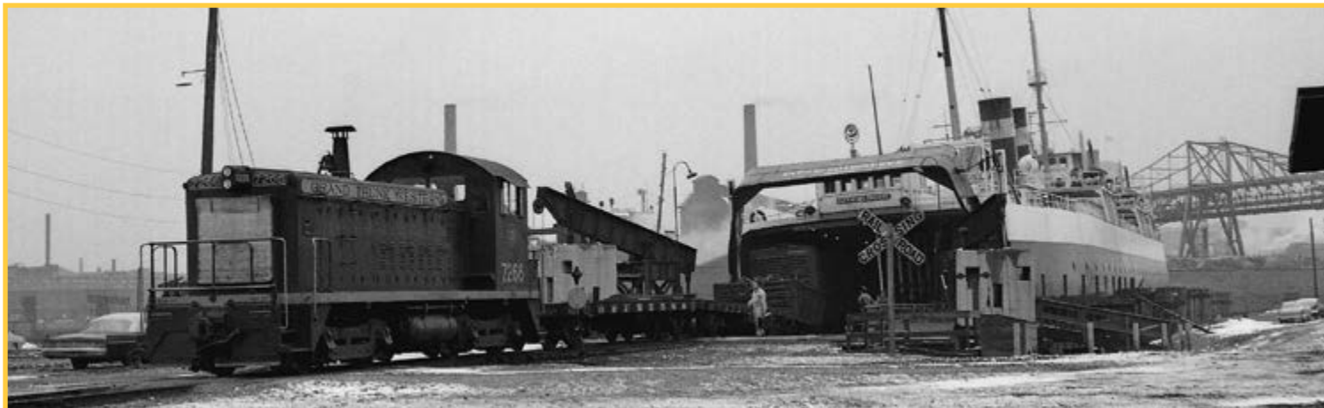
5. Below – Switching the outer track on the left, as we face it, on the City of Milwaukee . The reacher car is hooked onto a boxcar. In the background are facilities of the Milwaukee Solvay complex that burned coal into coke, making fuel gas in the process for the city's homes and industry. The coal unloading trestle is the skeletal structure on the right. Photo taken early 1965.
