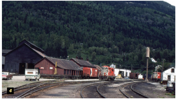
4 - The repair shops dominate in black. To the right, part of the adjoining white roundhouse is visible. The Tuscan red buildings (we called it "Revelstoke red", but also by a vulgar phrase) are stores. Two "Geeps" await assignment on the shop tracks. The elevated tank held sand for locomotives. It was dried in adjacent building and blown by compressed air up through a solid angled pipe. On cold nights it was a comfort to hold the warm filling pipe as it drained into loco storage tanks. Photo BW Williamson. was the former smithy. A coal forge, anvils, plus jigs and other tools of the metal trade seemed scattered about but must have been configured for efficiency when in use. In its earliest days other equipment would have included lathes, drill presses, power hammers, and milling machines. There being no electricity when it all was installed, power came indirectly from the steam plant. It would have mechanically driven line shafts (long axles) connected by bevelled gears at joints. These were all out of the way, but visible in the ceiling. Each shaft had on it flat pulleys (sheaves) over which broad, looped belts descended to individual machines on the shop floor. Operators could manually power a machine up or down with a hand lever which tightened its belt against the sheave, which in turn provided rotational power from the ever-spinning shaft.
