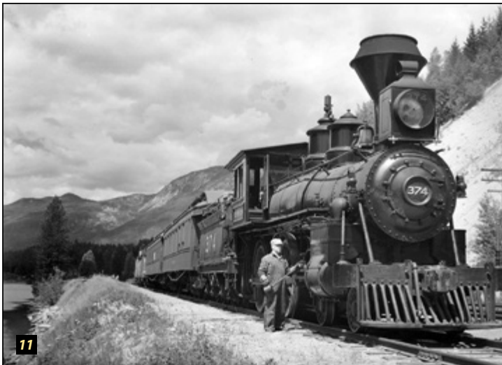
11 - Promotional photo from film Silent Barriers attributed to J. Sworbrick, somewhere near Three Valley Gap, BC. City of Vancouver Archives photo No. Can P88 N63. Men are identified as G. Leedham, engineer, and J. Johnson, fireman. The engine has been only cosmetically modified to appear as it did upon release from the factory.
