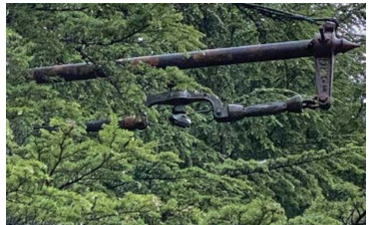
12. Detail of catenary support for pick up wire. Image by Rob Bryce, reproduced with permission.
