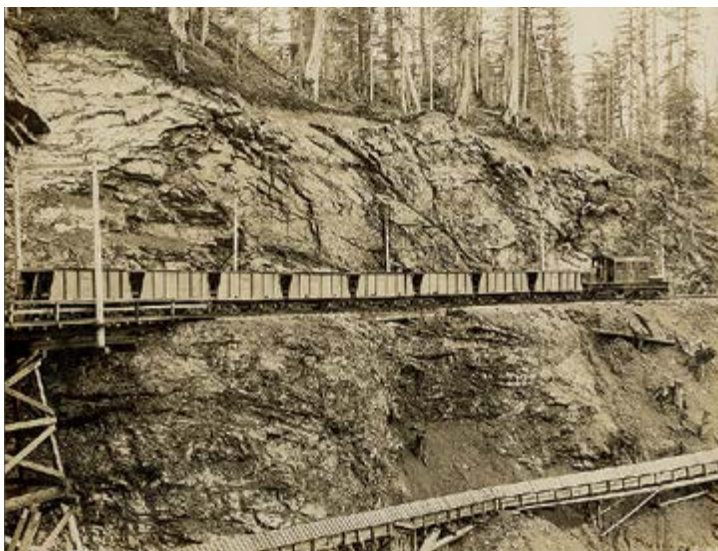
10. Steeple cab pulling standard eight-car train back to mine on the high line. Note the covered utility corridor lower down the cliff. Photograph reproduced by permission of UBC Archives (Accession Number BC1456-7-38).
