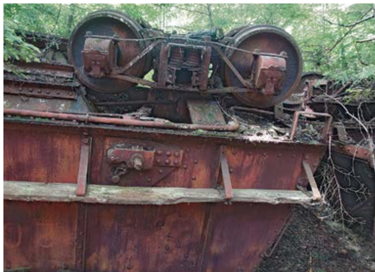
19. Bottom - One of three Anyox ore cars that were left upside down in the woods after a derailment. This shows the walkway that was only located on one side of the car and used by workers to access the car in winter to bar down (knock loose) frozen rock during the automated unloading process. Photo taken by the writer in June 2023.
