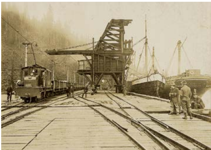
2. Dock view with steeple cab No. 11 on left track. The steam switcher, under the ore bin and the clam shell loaders, is switching the ore cars, loaded with flux, to the left hand track to add to the steeple cab's train. Photograph reproduced by permission of UBC Archives (Accession Number BC1456-7-54).
