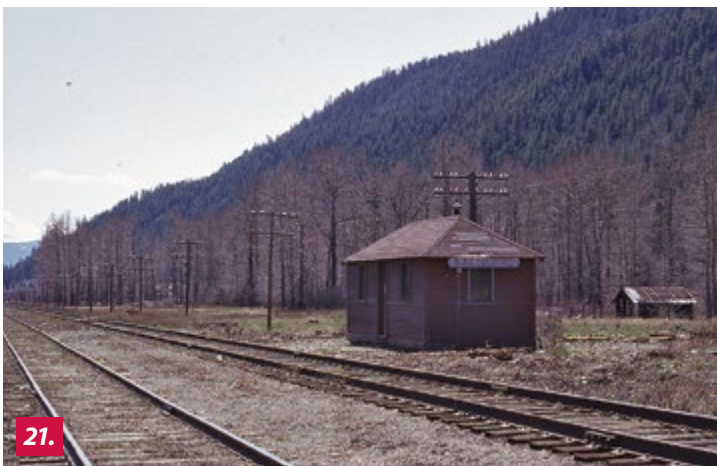
21. The view east towards the small shelter at Manning, April 28, 1974.
