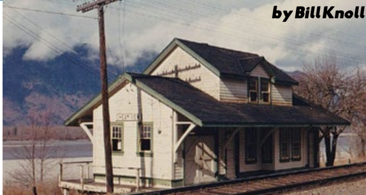
1. Cheam View Station. This mid-1960s image was recorded when the station, on the Canadian National line between Chilliwack and Hope, BC, remained active. The station was built in 1915 for about $2,000 by the CNoR as a Type C, combination station and section house. As built, the ground floor interior included a ticket office, a passenger waiting room and a freight shed. Also on the ground floor was accommodation for the agent's family including a living room, two bedrooms and a kitchen extending behind the station. The top floor had two bedrooms. Cheam View is on the Yale Subdivision at Mile Point 54.1. When I visited Cheam View station, it was a different setting, mist and gloom surrounded the station on the evening of June 28, 1971. Photo courtesy Mark Horne.
