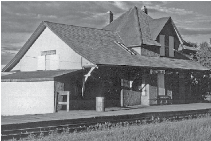
4. Delmas, Saskatchewan, at Mile Point 18.9 on CNRs Blackfoot Subdivision, is west of North Battleford. Its image was snapped in 1974. Delmas station was a Canadian Northern Railway standard third class building constructed to Plan 100-3. It was built in 1905 for $2963. Over several years the station received an addition to the original structure, had stucco applied to its exterior and eventually witnessed the installation of electricity. The station was demolished in 1982. Photo by Bill Knoll.
