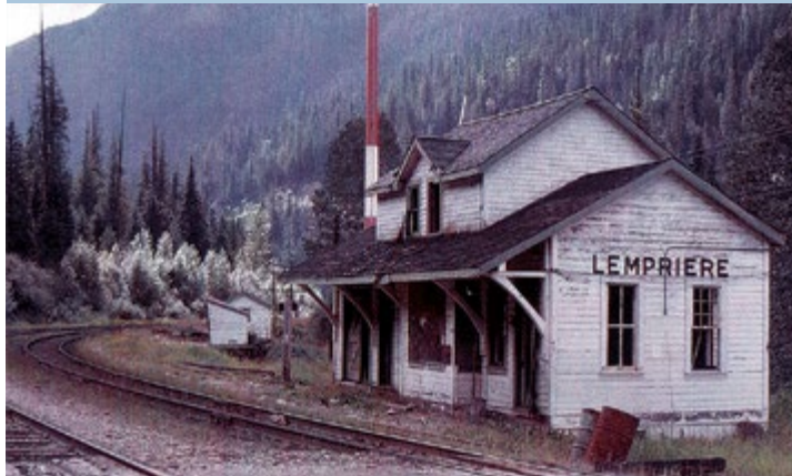
2. Lempriere Station was a CNoR combination station and section house, Type C, built to CNoR Plans 100-47 and 100-98. When I visited the site, the station was standing on timber cribs, apparently being prepared for removal to somewhere else. However, the station was demolished in 1973. Photo by Stan Styles, Les Kozma collection.
