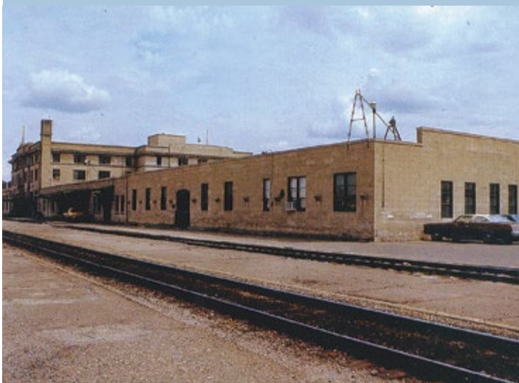
5. Track side of the CPR station in Regina. Photo by Bill Knoll.
